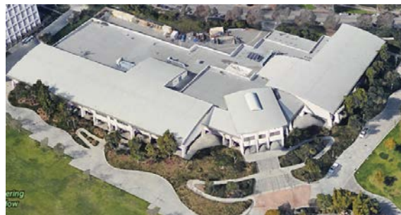
Figure 1 – California State Polytechnic University, Pomona Engineering Building
