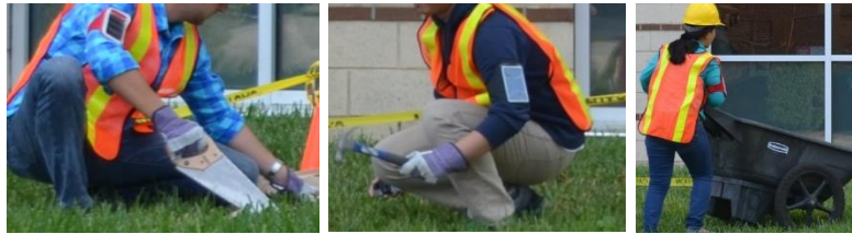
Figure 4: Worker performing activities in 3 categories with data collection device (i.e. smartphones) affixed on their arms
